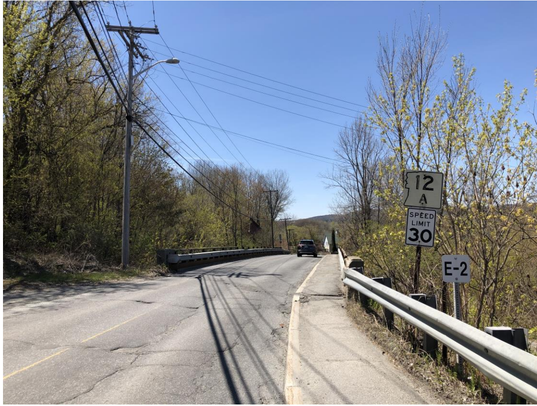
Rte 12A/So Main Street Bridge
