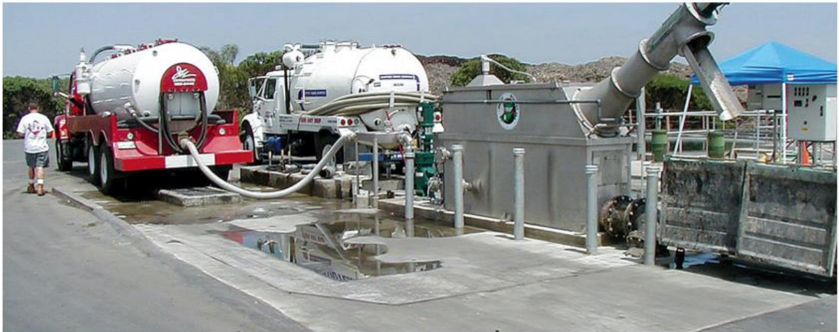
Proposed Septage Receiving Facility
