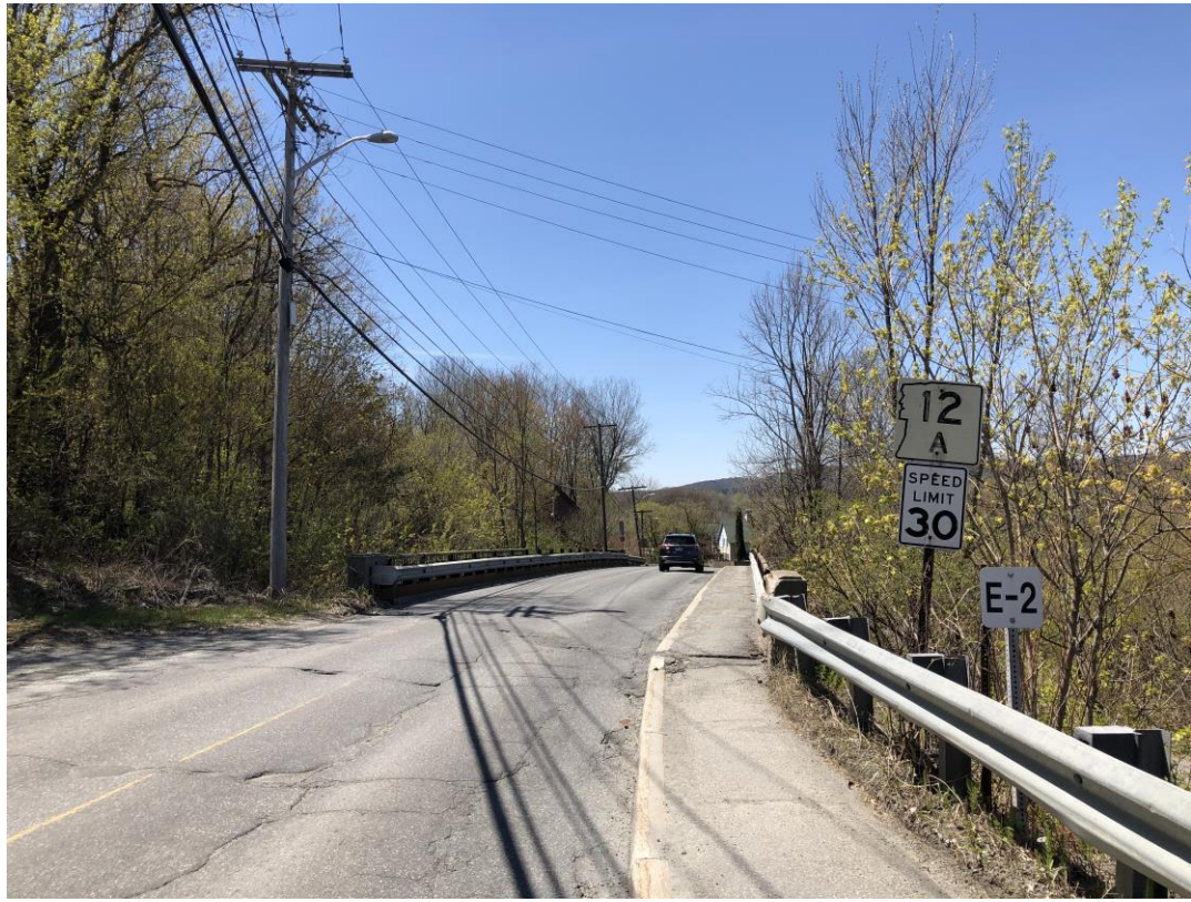
Rte 12A/So Main Street Bridge
