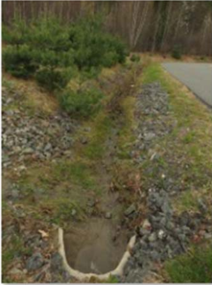
(11) 2019_05_01 outflow ditch near access road beginning
