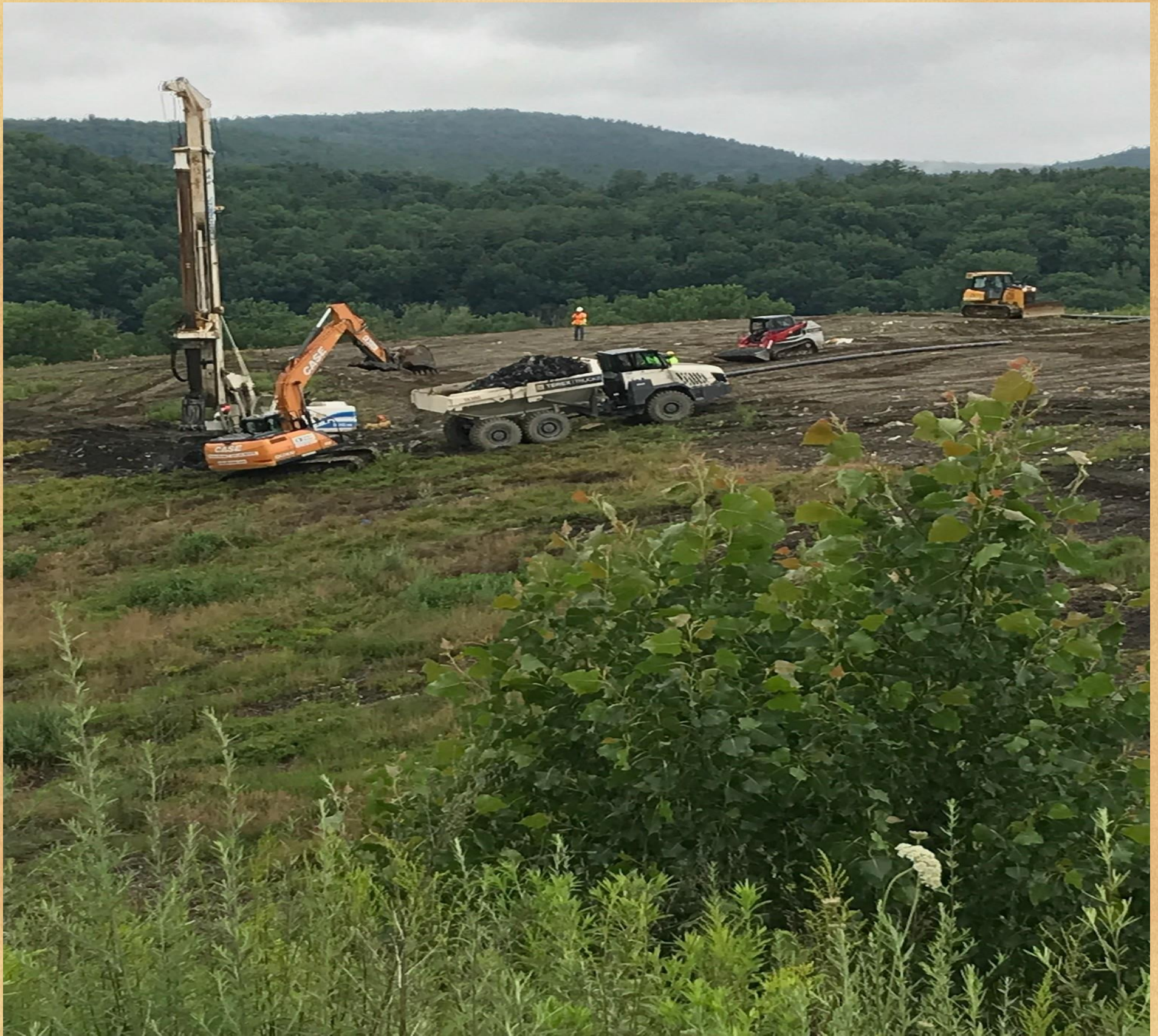
Installation of Gas Collection - Summer 2021
