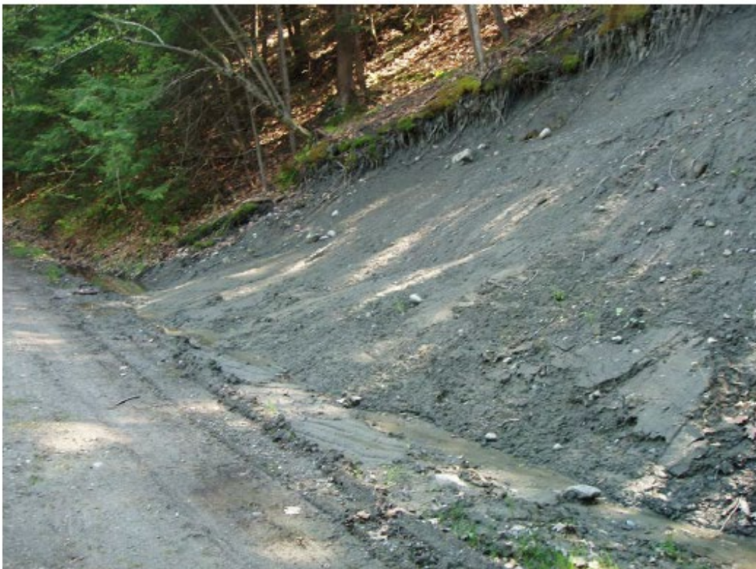
Cleaned Failed Uphill Slope at Site #2
