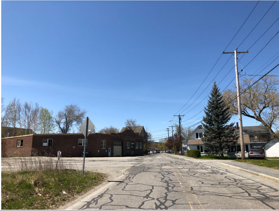
Spencer Street Existing Conditions
