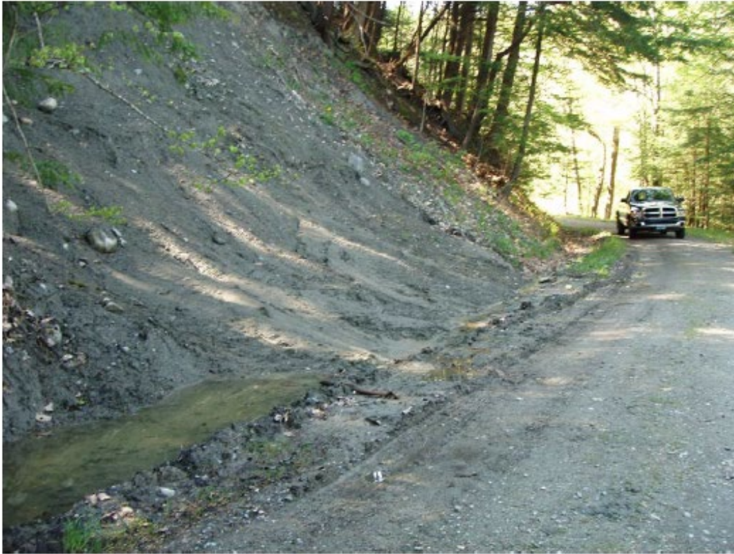
Cleaned Failed Uphill Slope at Site #2
