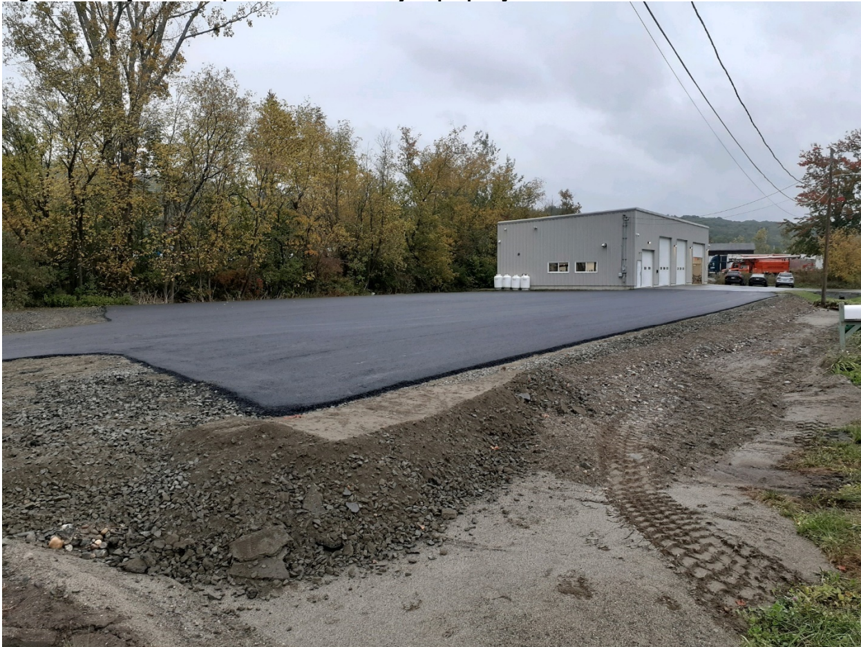
Figure 3. Newly installed pavement at the subject property.
