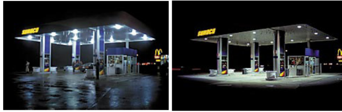
The above photographs illustrate the impact of glare on a lighting installation. The left photo has high-glare, non-recessed fixtures under the canopy. Note how bright the lights themselves are and how dark the pump area is. The right photo shows the same gas station canopy with full-cutoff, recessed fixtures. Note how the light is directed effectively toward the gas pumps. Images from http://www.skyandtelescope.com
