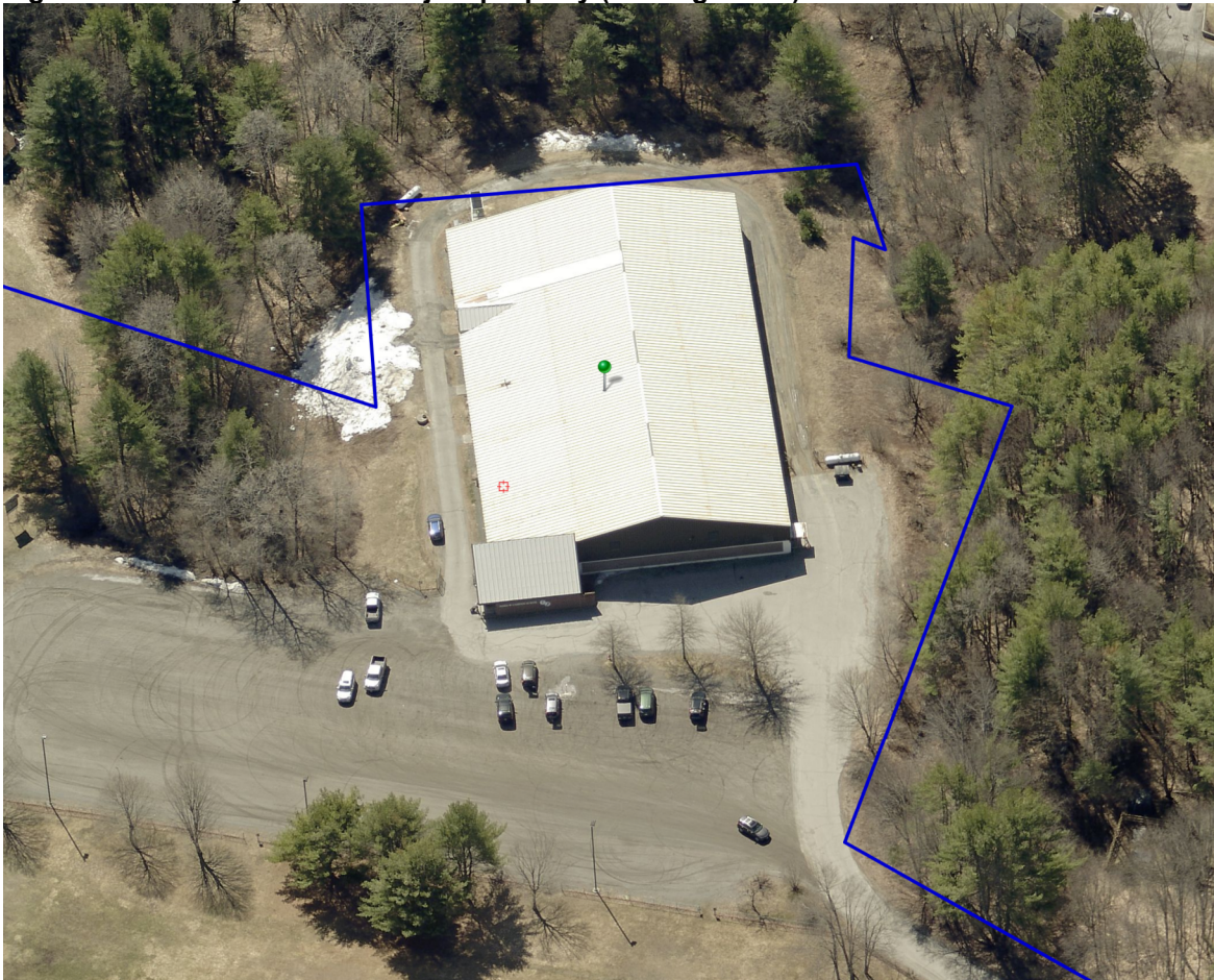
Figure 3. Bird's Eye View of subject property (looking south).
