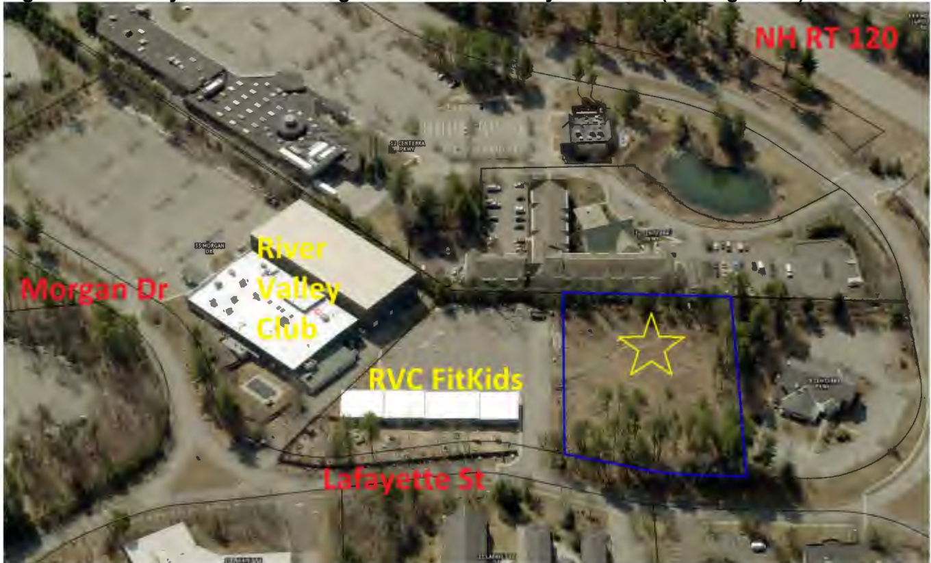
Figure 1. Bird's Eye View of 33 Morgan Drive and 12 Lafayette Street (looking south).
