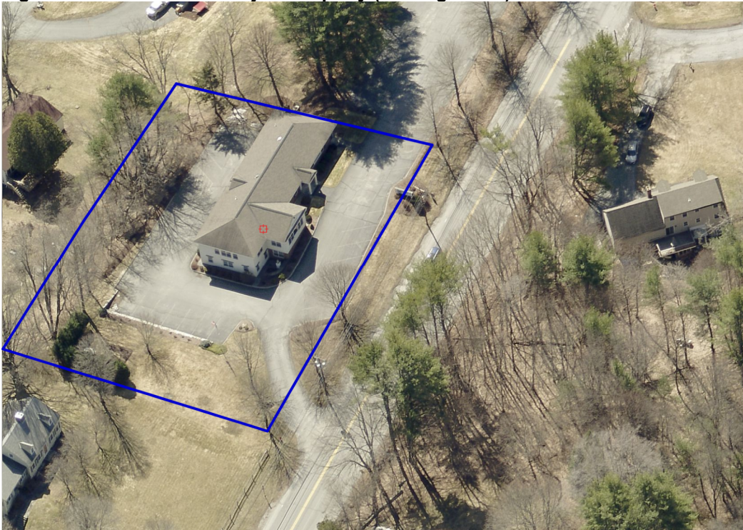
Figure 1. Aerial View of Subject Property (looking south).
