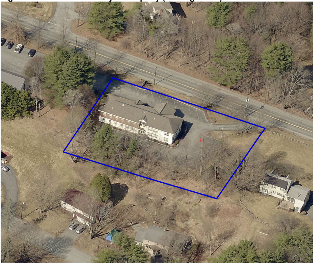
Figure 1. Aerial View of Subject Property (looking south).
