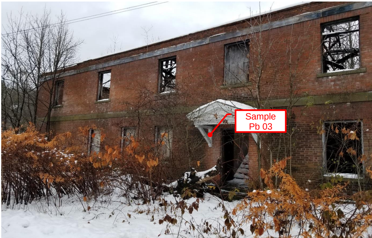
Photograph 12: Bunk House – Exterior 1st Floor Paint on Wood Threshold. Blue Paint Chips (Lead, 31.9 mg/Kg, Both Entrances)
