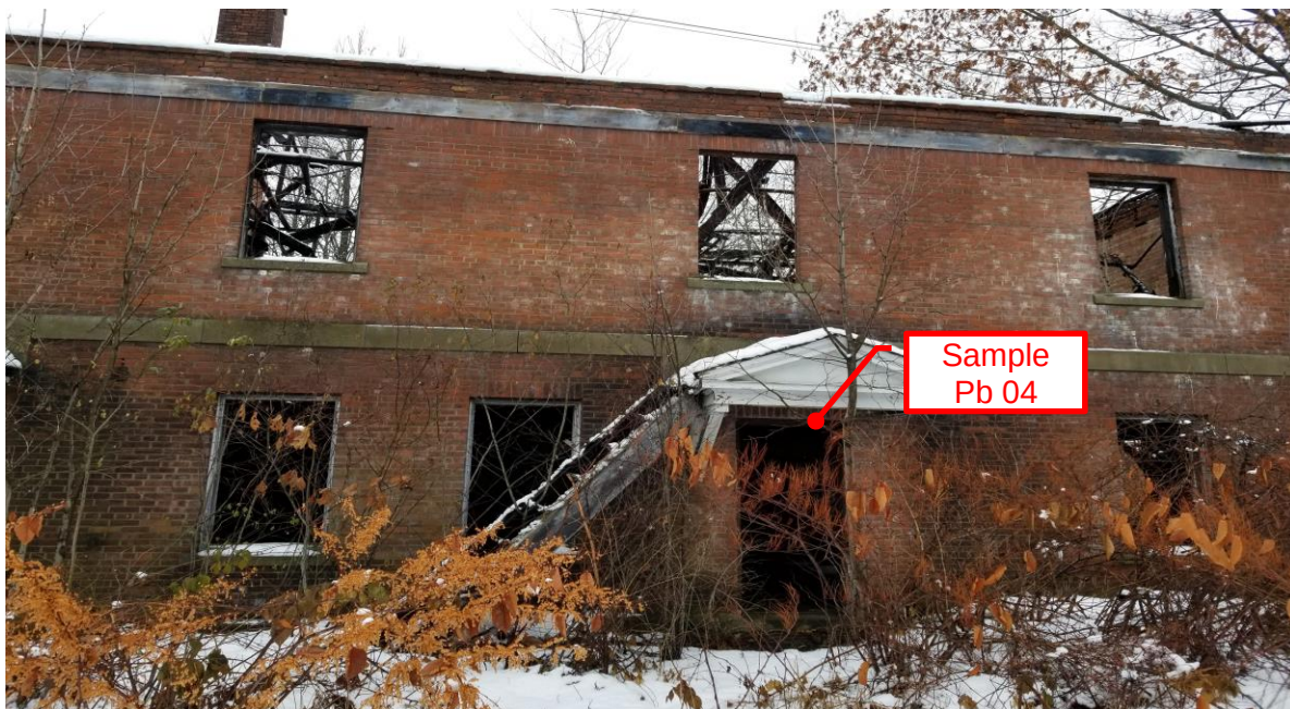
Photograph 12: Bunk House – Exterior 1st Floor Paint on Wood Threshold. Blue Paint Chips (Lead, 31.9 mg/Kg, Both Entrances)
