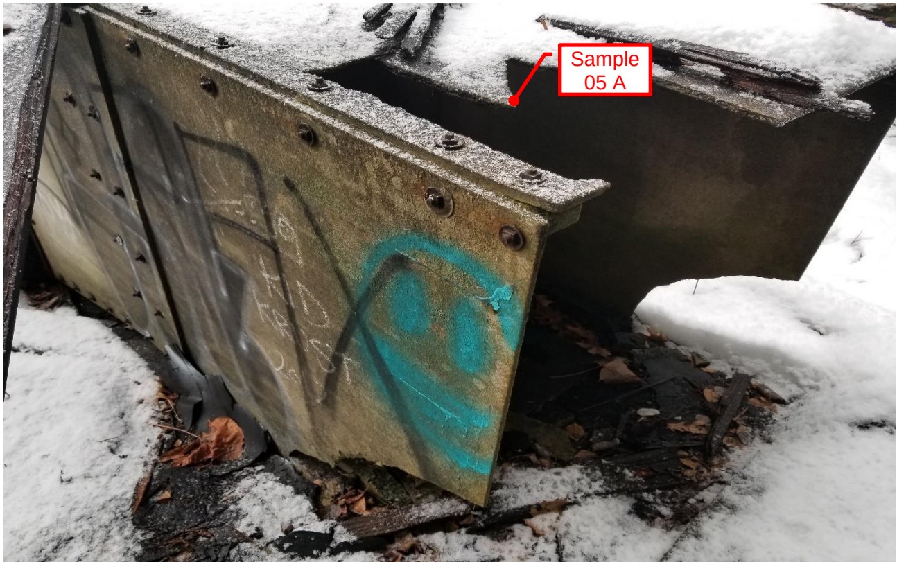
Photograph 4: Round House – Roof Chute. Cementitious Chute Board (ACM, 20% Chrysotile, 400 SF each – 9 Total Chutes)
