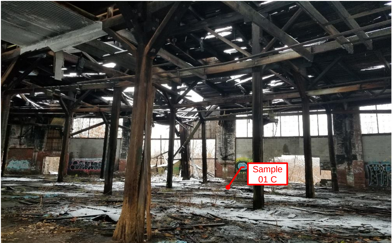
Photograph 2: Round House – East Wall. Black Built-Up Roofing Material (ACM, 25% Chrysotile)
