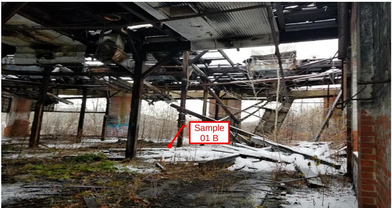
Photograph 2: Round House – East Wall. Black Built-Up Roofing Material (ACM, 25% Chrysotile)
