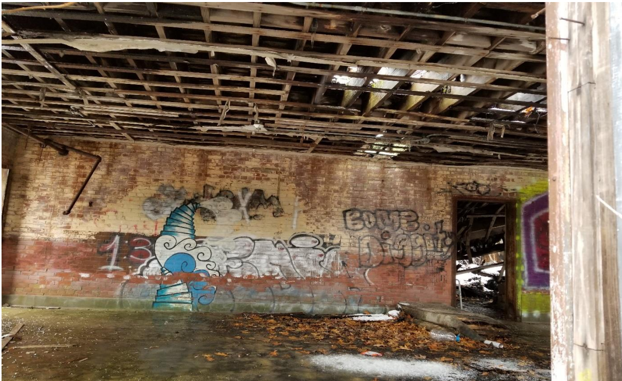
Photograph 10: Bunk House – Interior 1st Floor Paint on Brick Walls. Green Paint Chips (Lead, .30 mg/Kg, All Walls)
