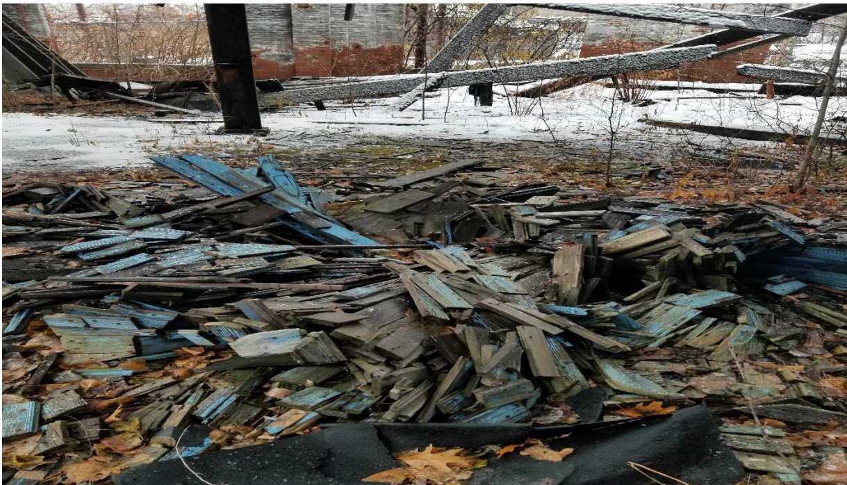
Photograph 8: Round House – Wood Debris on Floor. Blue Paint Chips (Lead, 1.34 mg/Kg, 1 CY - 2 Debris Piles)
