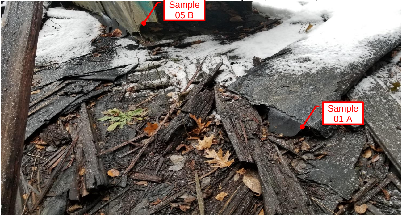
Photograph 4: Round House – Roof Chute. Cementitious Chute Board (ACM, 20% Chrysotile, 400 SF each – 9 Total Chutes)
