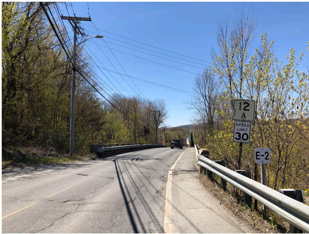
Rte 12A/So Main Street Bridge
