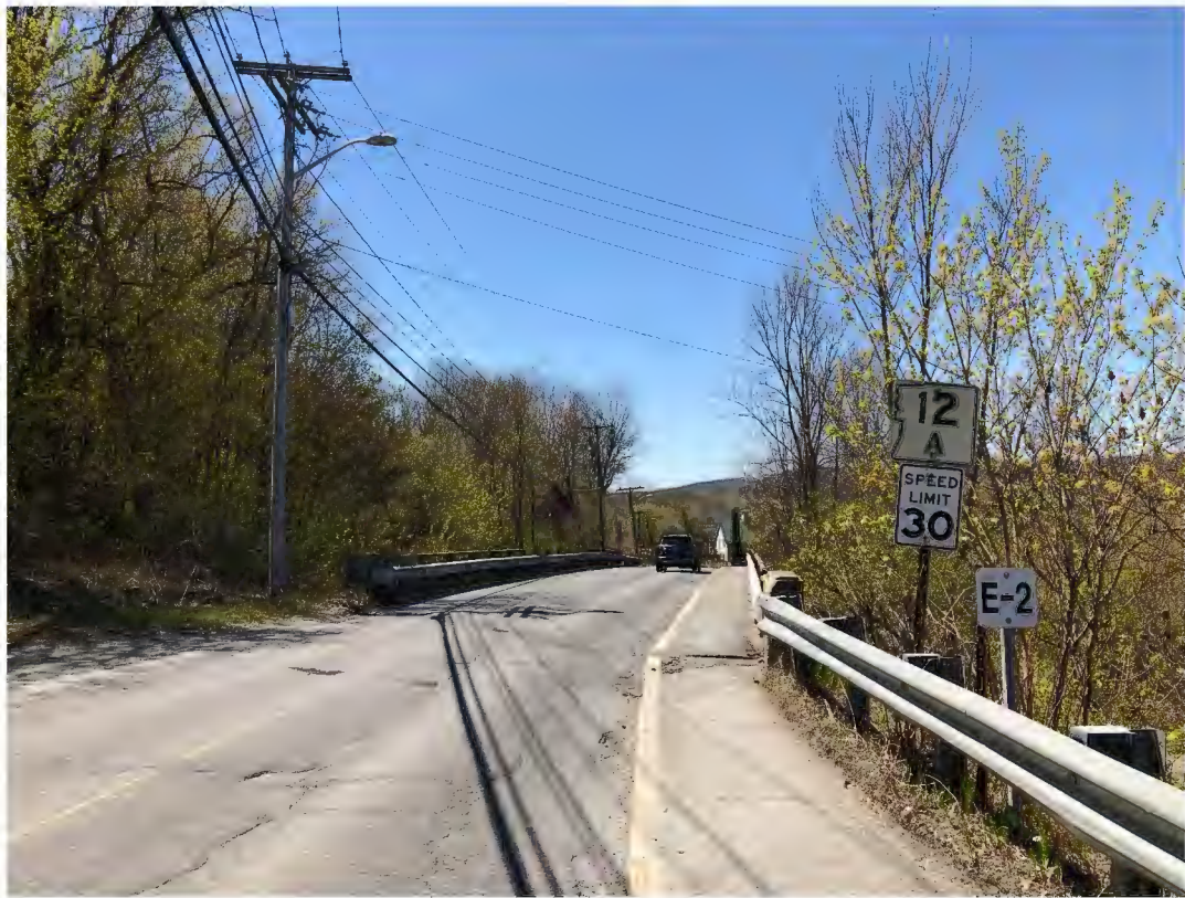
Rte 12A/So Main Street Bridge
