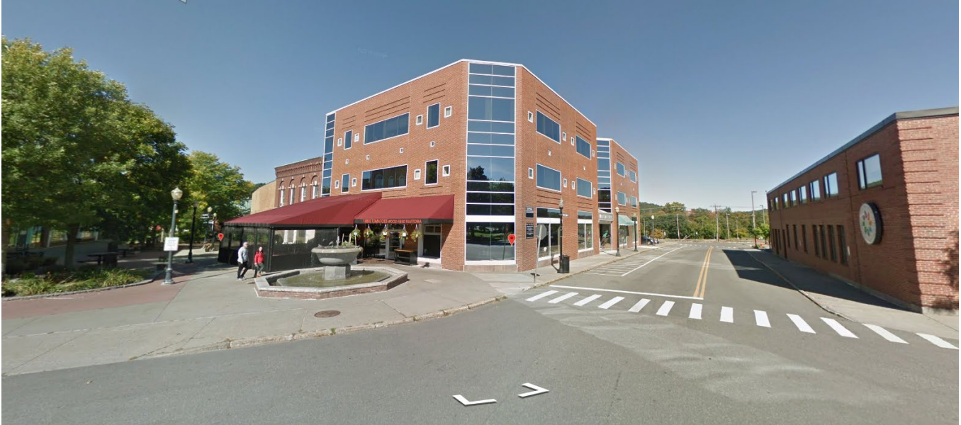
Figure 1. Street view of property.
