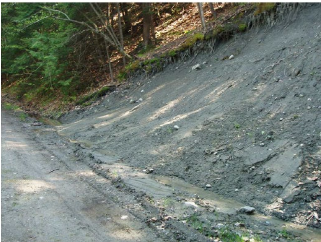
Cleaned Failed Uphill Slope at Site #2
