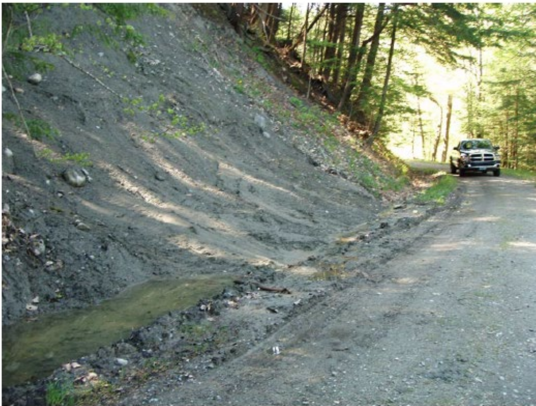
Cleaned Failed Uphill Slope at Site #2
