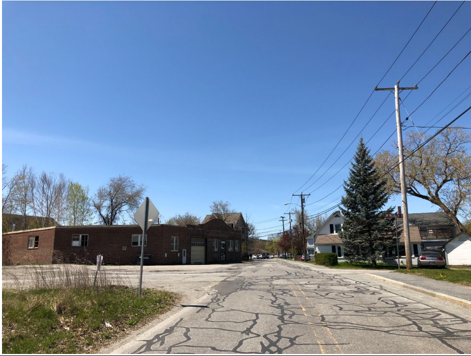
Spencer Street Existing Conditions
