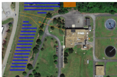
City of Concord Fire Station, Waste Water Treatment Plant 720 kW (2015-20)
