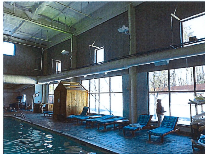
POOL 101 NORTH EXTERIOR WALL
