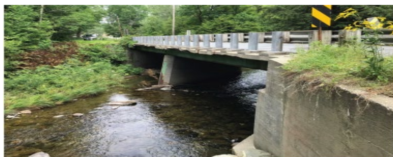
26 27 Trues Brook Road 28 Bridge
