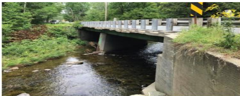
Trues Brook Road Bridge
