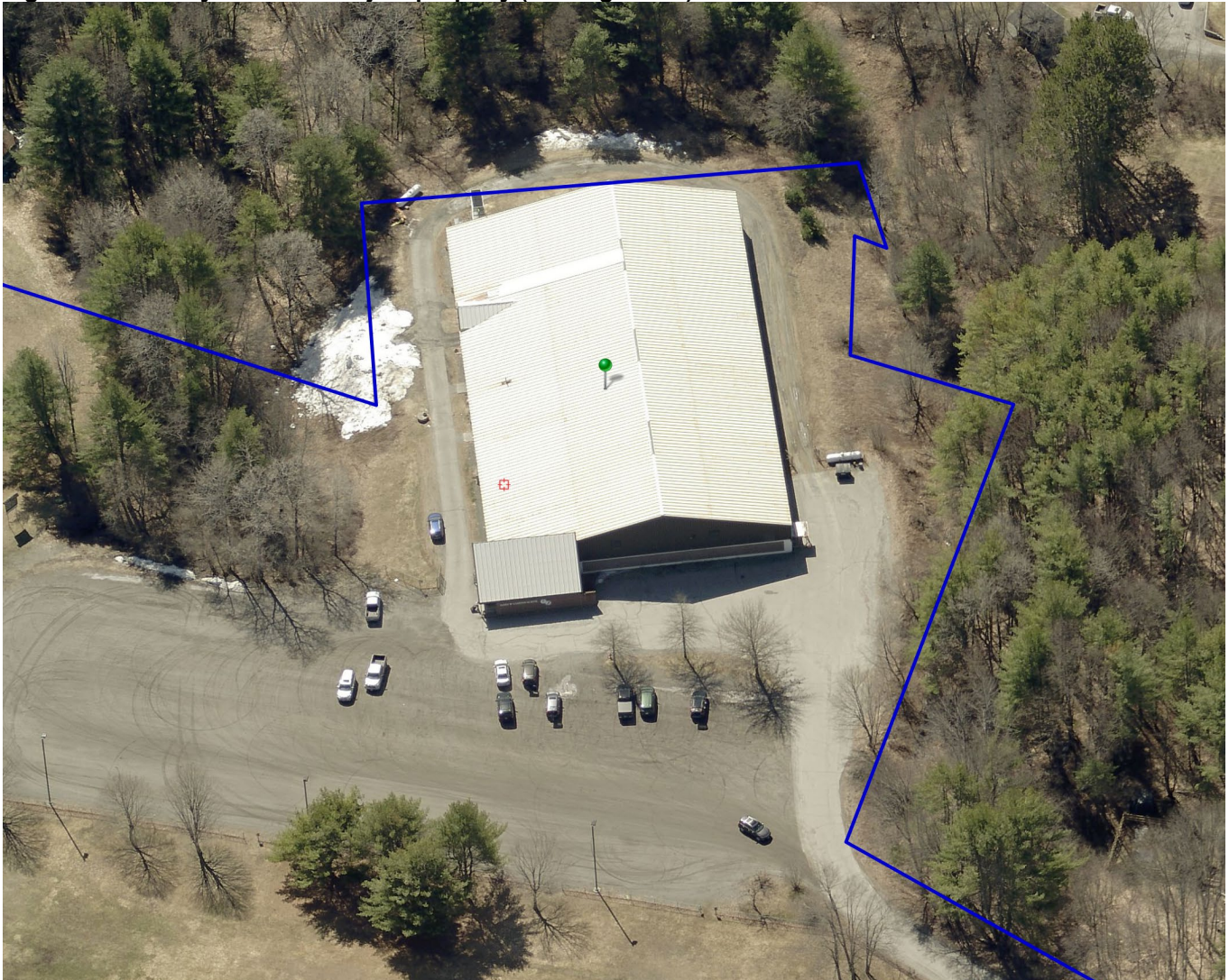
Figure 3. Bird's Eye View of subject property (looking south).
