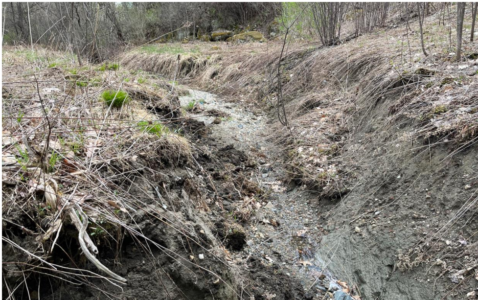
Image 2: Erosion Gully (Looking East)
