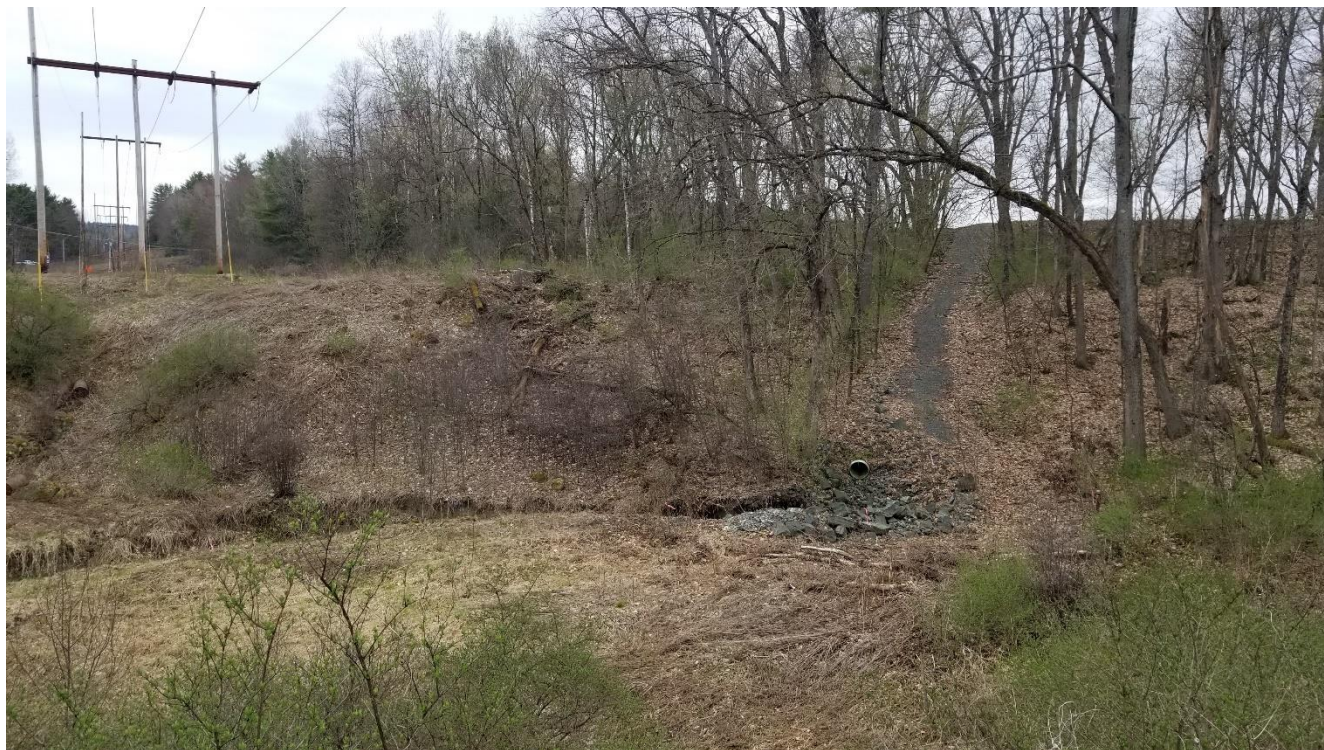
Photo 1. LW1 outfall overview from trail.
