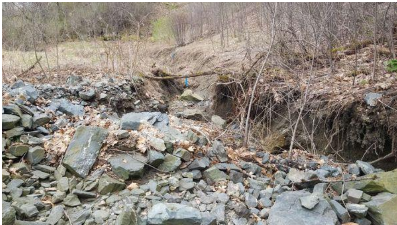
Photo 10. LS2 at outfall.
