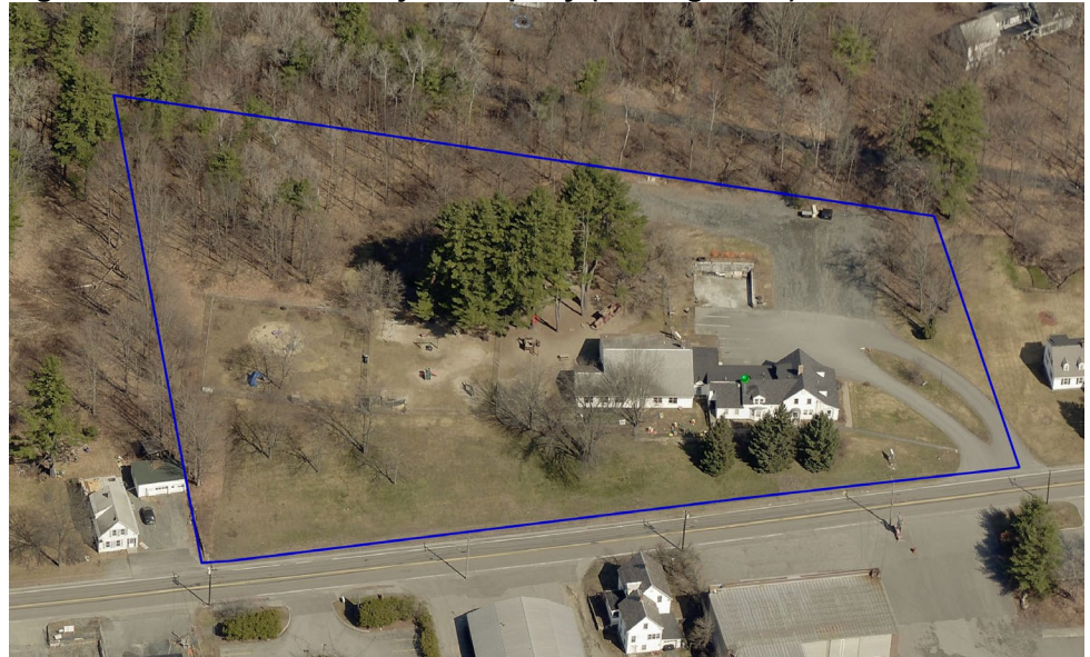
Figure 1. Aerial View of Subject Property (looking north).
