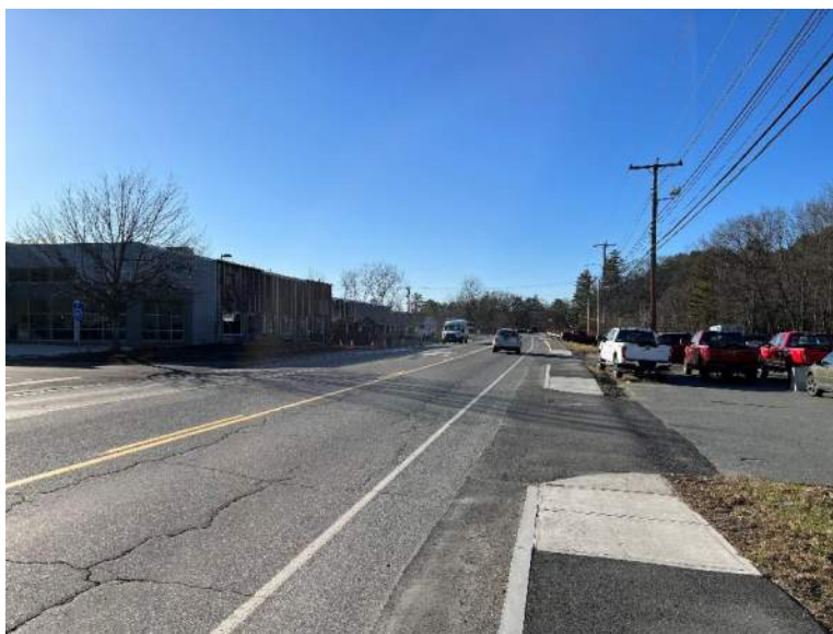
Figure 6 - Ford Dealership Under Construction
