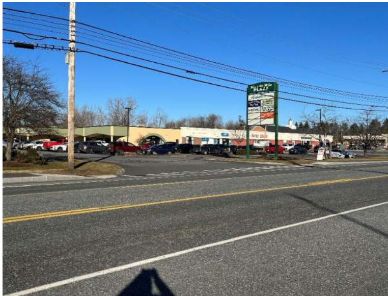
Figure 7 - Miracle Mile Plaza Western Driveway
