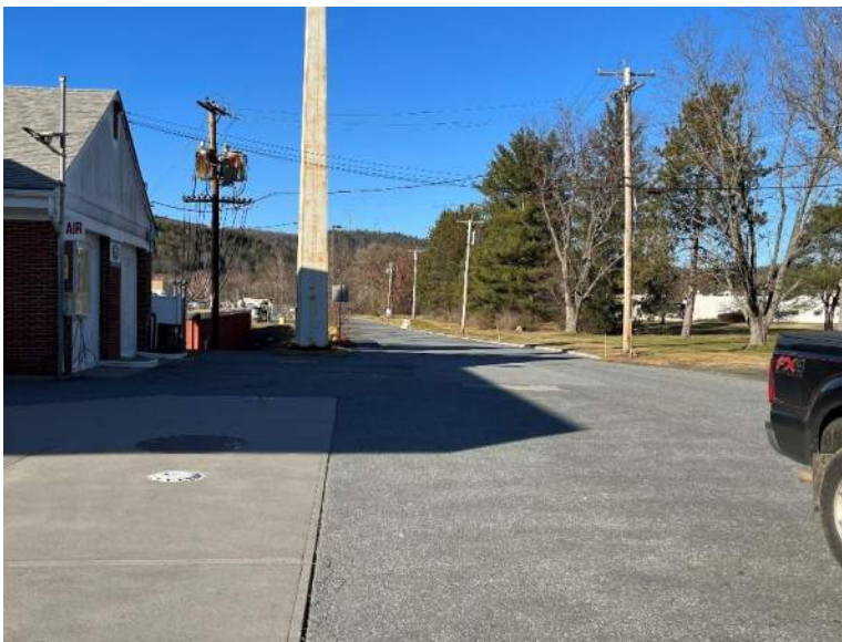
Figure 12 - End of Sidewalk in Tractor Supply Driveway
