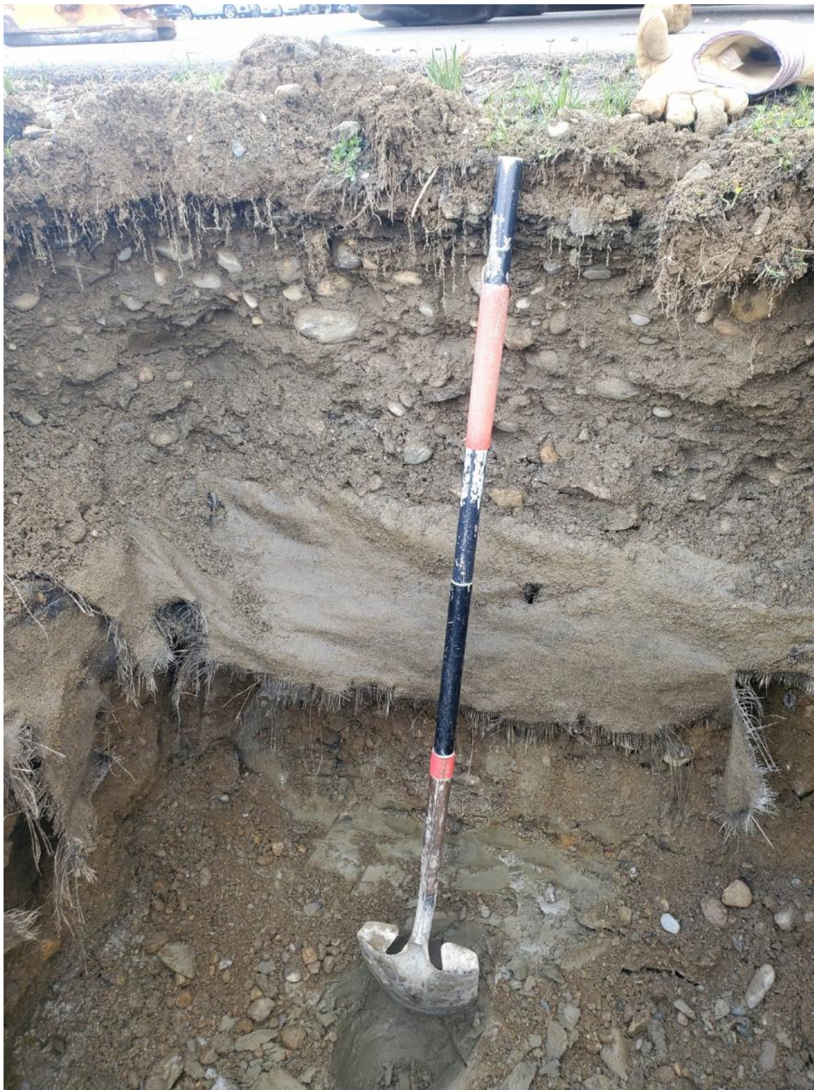
Soil conditions at TP-2, edge of pavement
