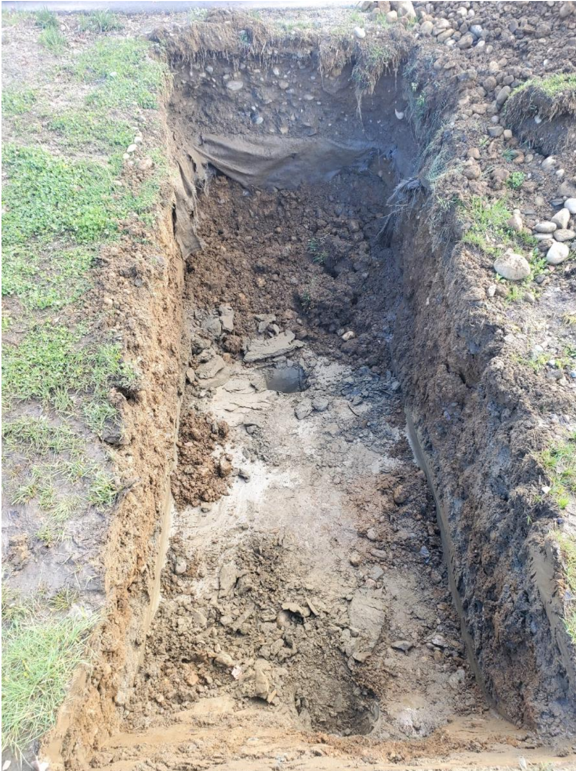
Measurement point TP-1 reflected in shovel hole in foreground. Note water on ground surface of grass swale.
