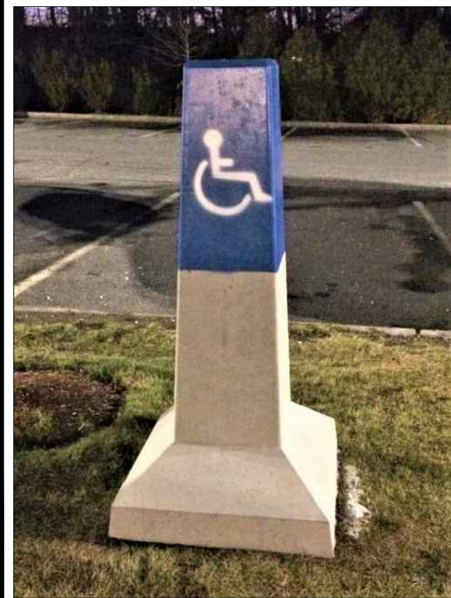
C18 MOVEABLE CONCRETE BOLLARDS WITH PAINTED ADA SYMBOL.
