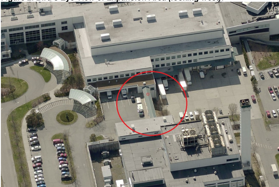
Figure 2. Bird's Eye View of Expansion Area (looking west).
