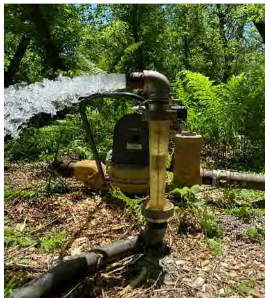
Short Term Pumping Test on TW 1-21
