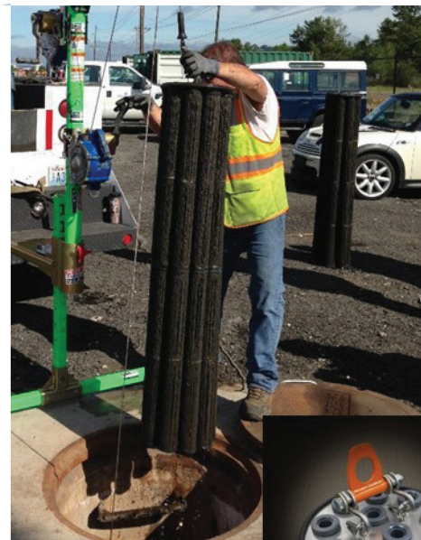
Cartridge Removal & Lifting Device
