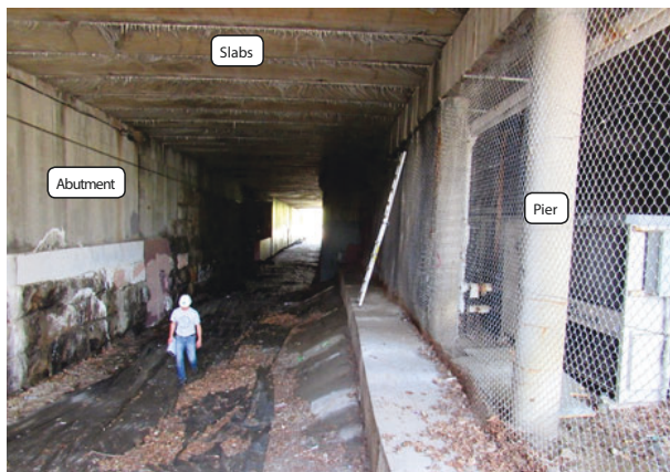
TUNNEL STRUCTURAL COMPONENTS
