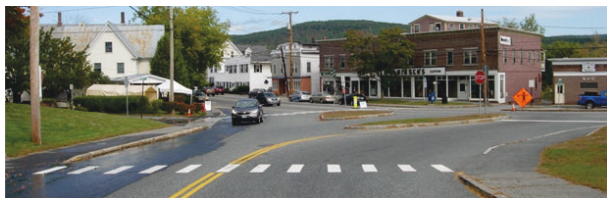
HIGH STREET NORTHBOUND APPROACH AT HANOVER STREET – LONG CROSSWALK ON HANOVER STREET & NUMEROUS CURB-CUTS.
