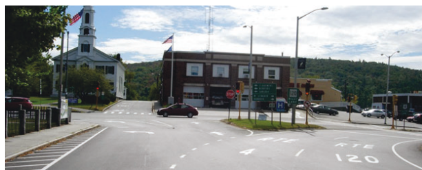
SOUTHBOUND APPROACH OF WEST PARK STREET AT THE INTERSECTION OF CHURCH STREET/FIRE STATION AND HANOVER STREET.
