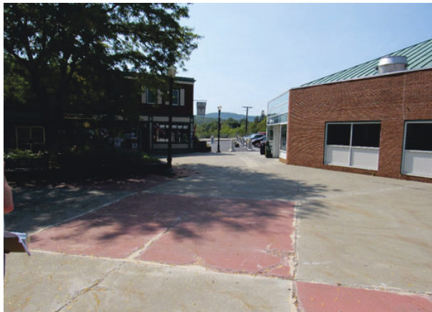
PLAZA AREA ABOVE THE TUNNEL
