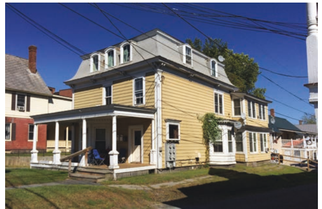
Residential building on Hanover Street
