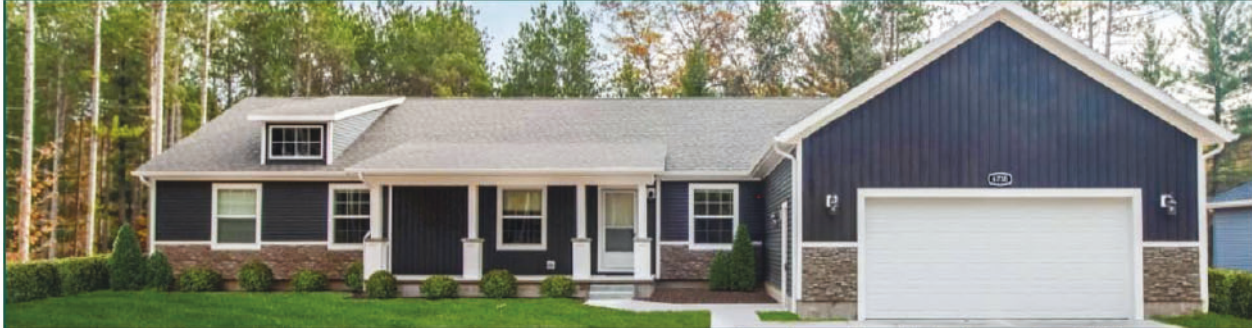
Example of a "CrossMod" single family residence where a portion of the home is stick-built on site which meets the State Building Code, and a portion of the house is built at an off-site facility which meets HUD housing code.
