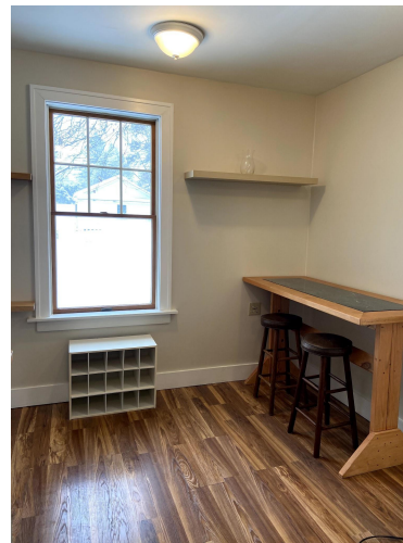
Added a second means of egress & kitchen. Electricians did electrical work and a plumber did the sink plumbing.
