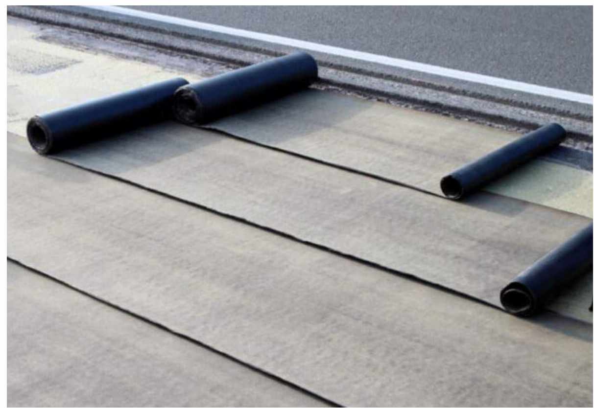
EPDM RUBBER ROOFING SYSTEM - TYPICAL AT ROOF.
