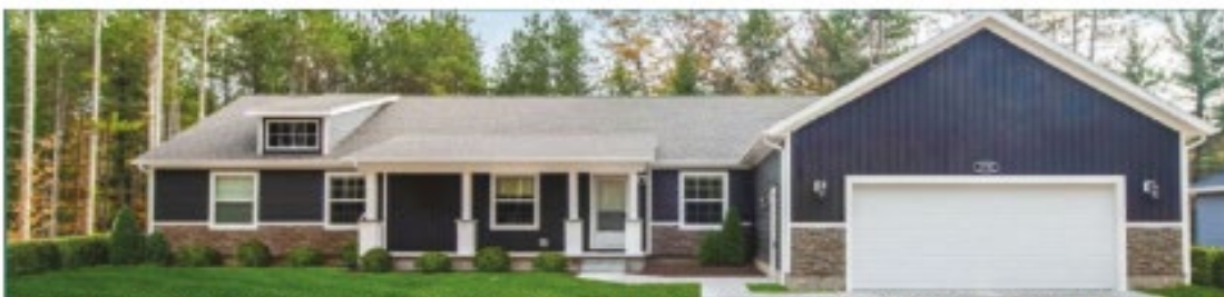
Example of a "CrossMod" single family residence where a portion of the home is stick-built on site which meets the State Building Code, and a portion of the house is built at an off-site facility which meets HUD housing code.
