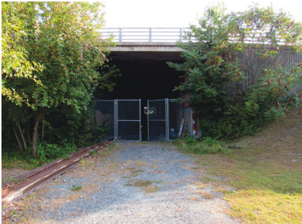
THE TUNNEL IS CLOSED WITH A CHAIN LINK FENCE
