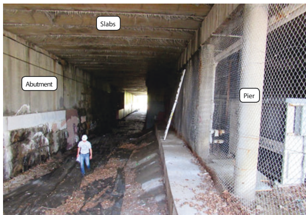
TUNNEL STRUCTURAL COMPONENTS
