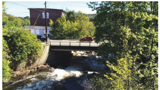
MASCOMA RIVER BRIDGE CROSSING
