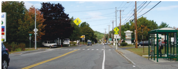
COVERED BUS SHELTER ON HANOVER STREET & PEDESTRIAN CROSSING WITH NON-FUNCTIONING PEDESTRIAN CALL BUTTONS.
