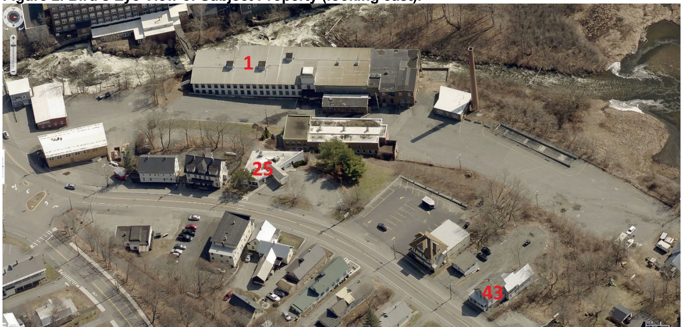
Figure 2. Bird’s Eye View of Subject Property (looking east).
