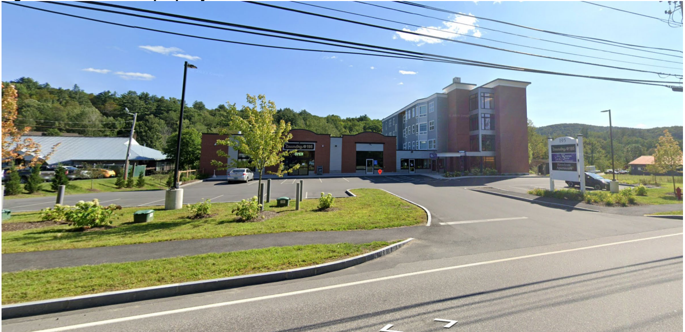
Figure 1. Street view of property.
