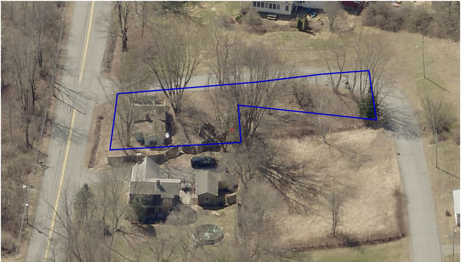
Figure 1. Bird's Eye View of subject property (looking south) prior to the demolition of the previous structure and the construction of the new home.
