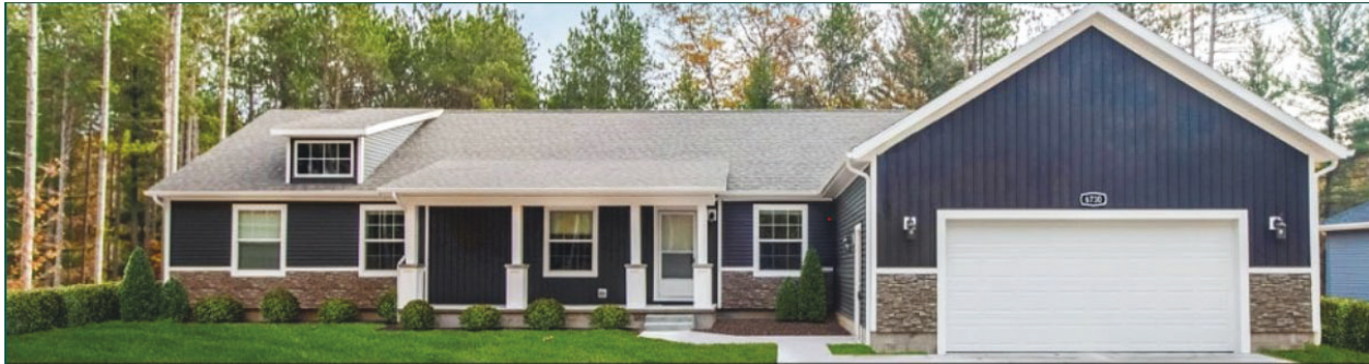
Example of a "CrossMod" single family residence where a portion of the home is stick-built on site which meets the State Building Code, and a portion of the house is built at an off-site facility which meets HUD housing code.
