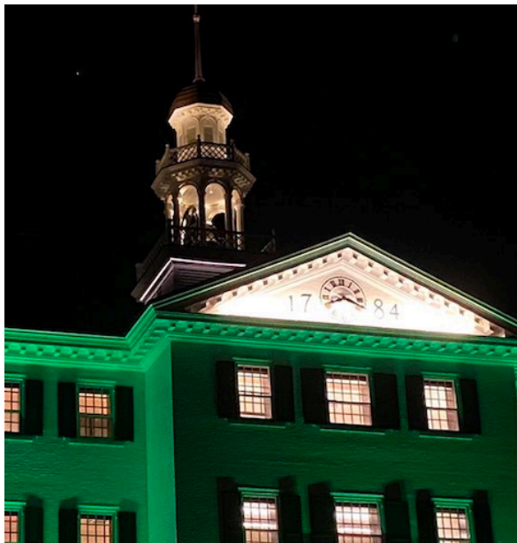
Floppy flex lighting on bell tower base
