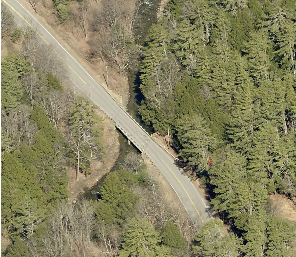
Figure 2. Bird's Eye View of Existing Bridge (looking north)
