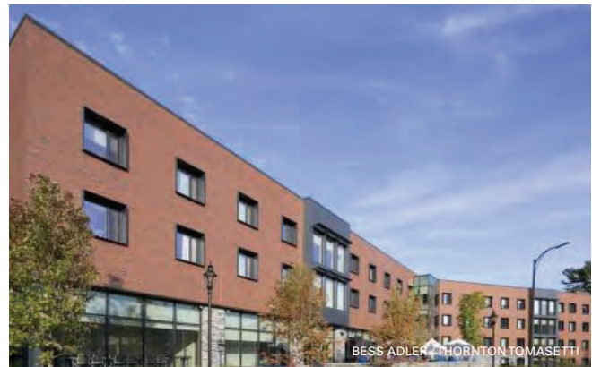
Pine Hall, at Wheaton College, is the first Phius+ certified residence hall in Massachusetts. (Phius+2015)
