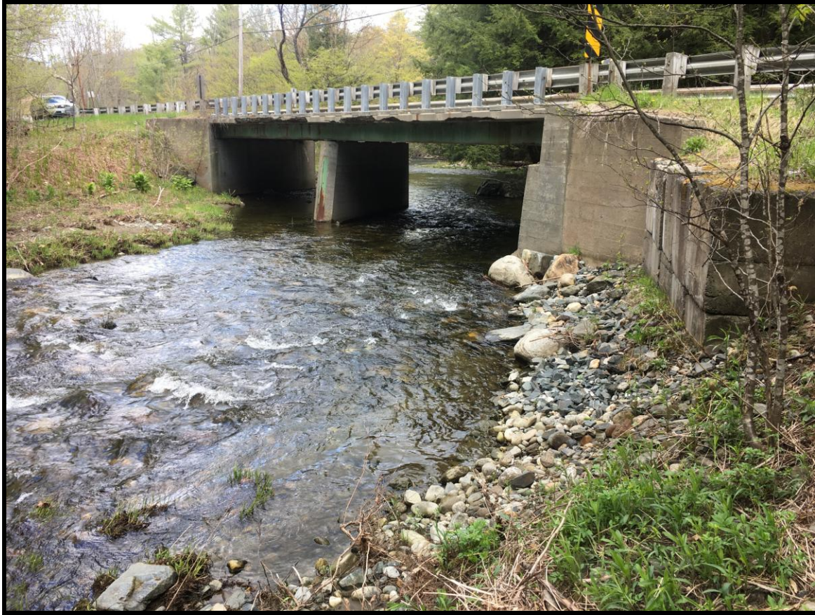
General view of Wetland A looking downstream (north) at proposed project location.
