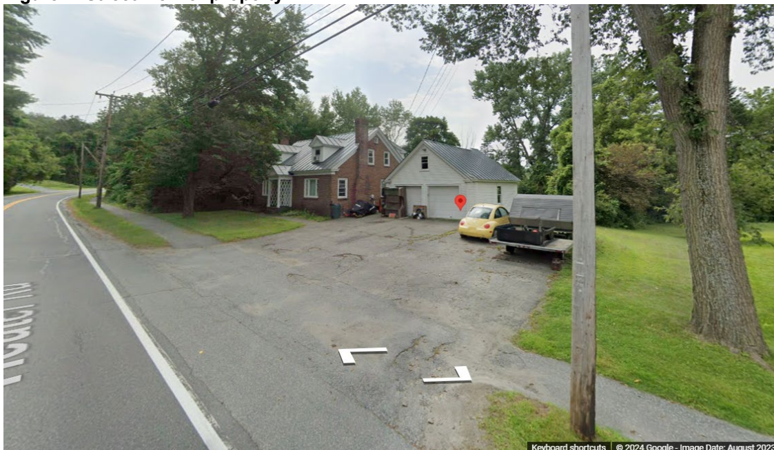
Figure 1. Street view of property.
