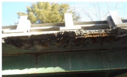
Underside of Bridge Deck
