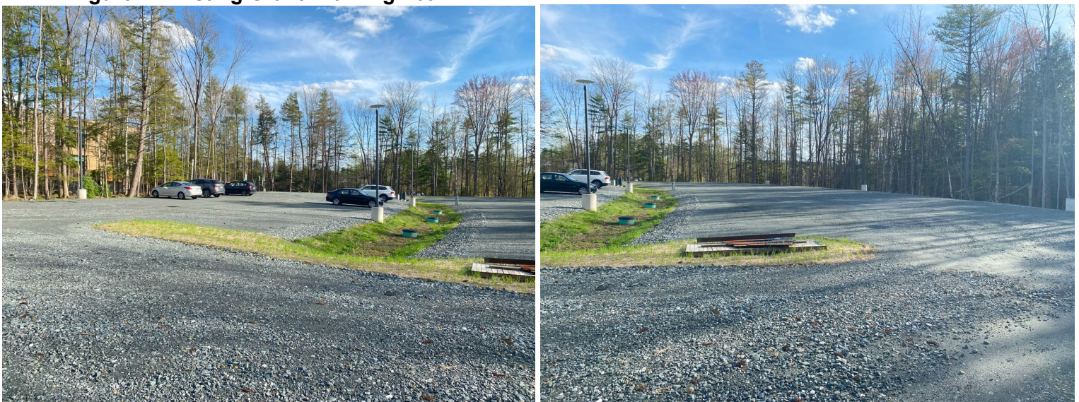
Figure 1. Existing Gravel Parking Lot.
