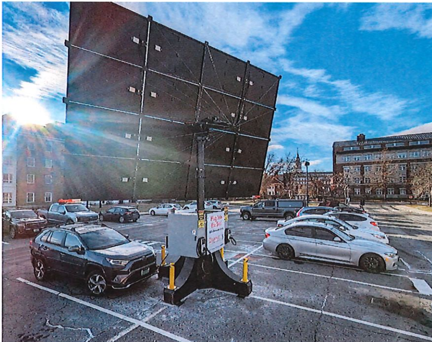
Solar EV Charger, Dartmouth College
