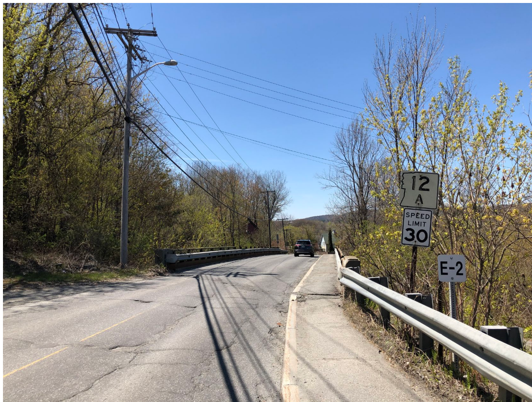
Rte 12A/So Main Street Bridge
