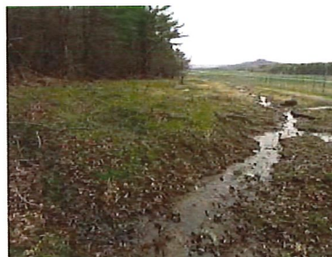
File Name : 2019_05_01 (11) begin open ditch again to N.JPG
