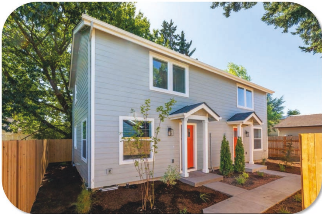
Figure 12: A newly constructed backyard duplex project that retained and fixed up the front house.
