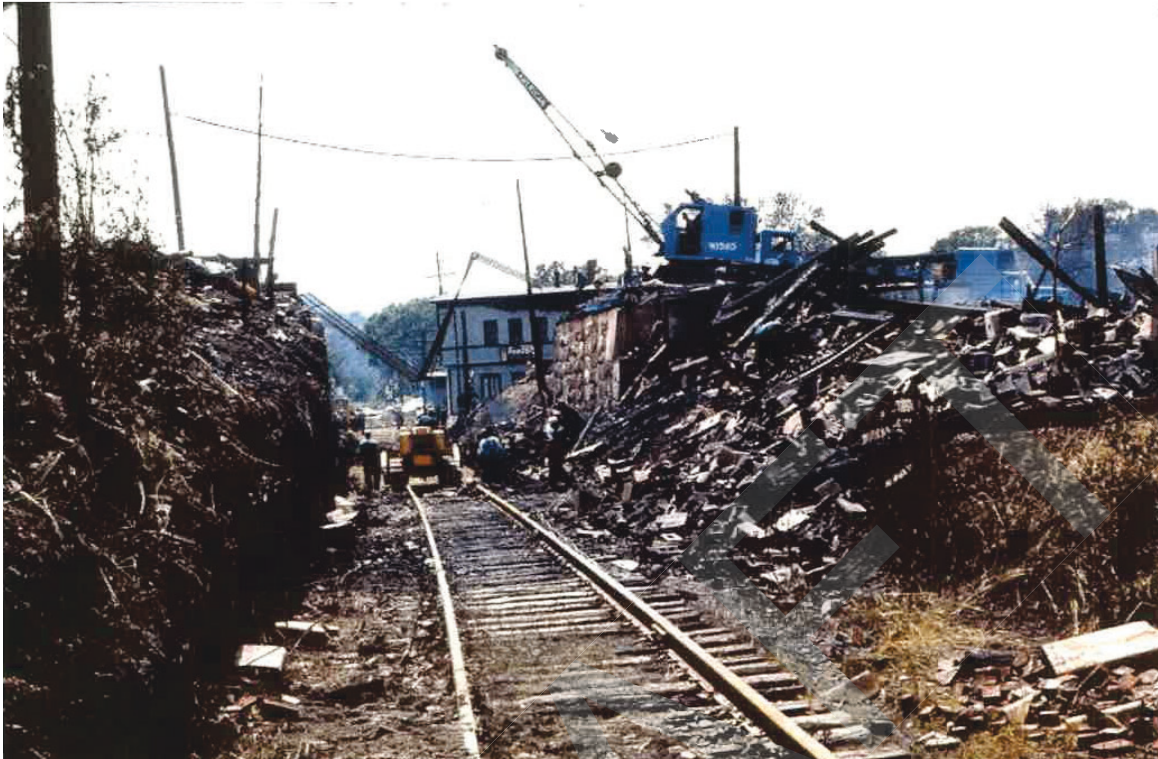
VIEW ALONG THE RAIL LINE SHOWING DESTRUCTION OF THE 1964 FIRE SOURCE: VALLEY NEWS
