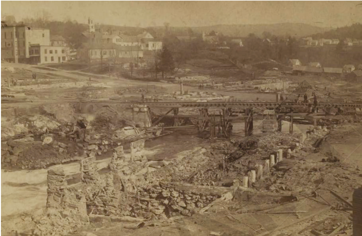
1887 - VIEW SOUTHEAST FROM HIGH STREET SHOWING DESTRUCTION OF THE 1887 FIRE SOURCE: NH HISTORIC SOCIETY
