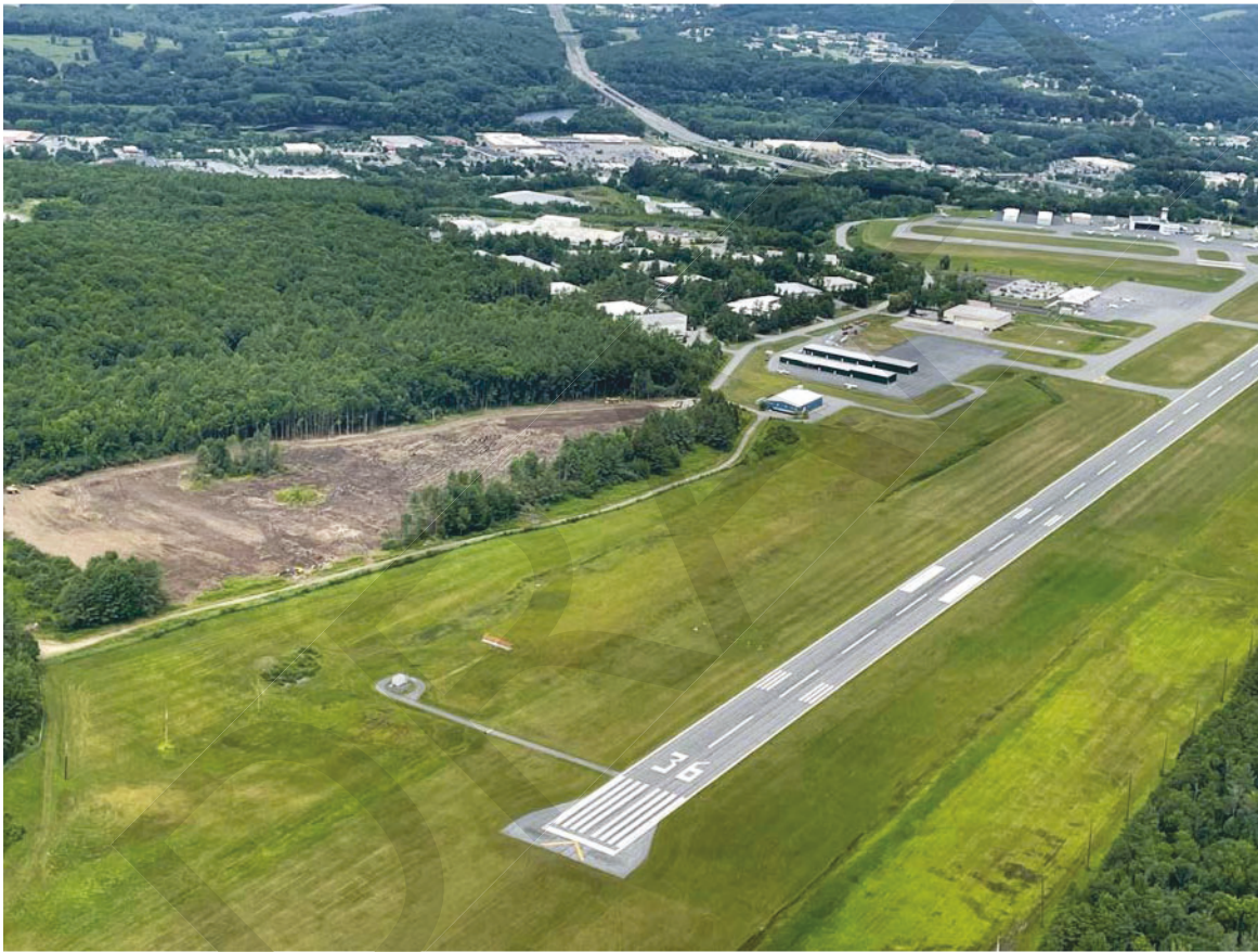
LEBANON MUNICIPAL AIRPORT (APPROXIMATELY 2 MILES FROM PROJECT SITE)
