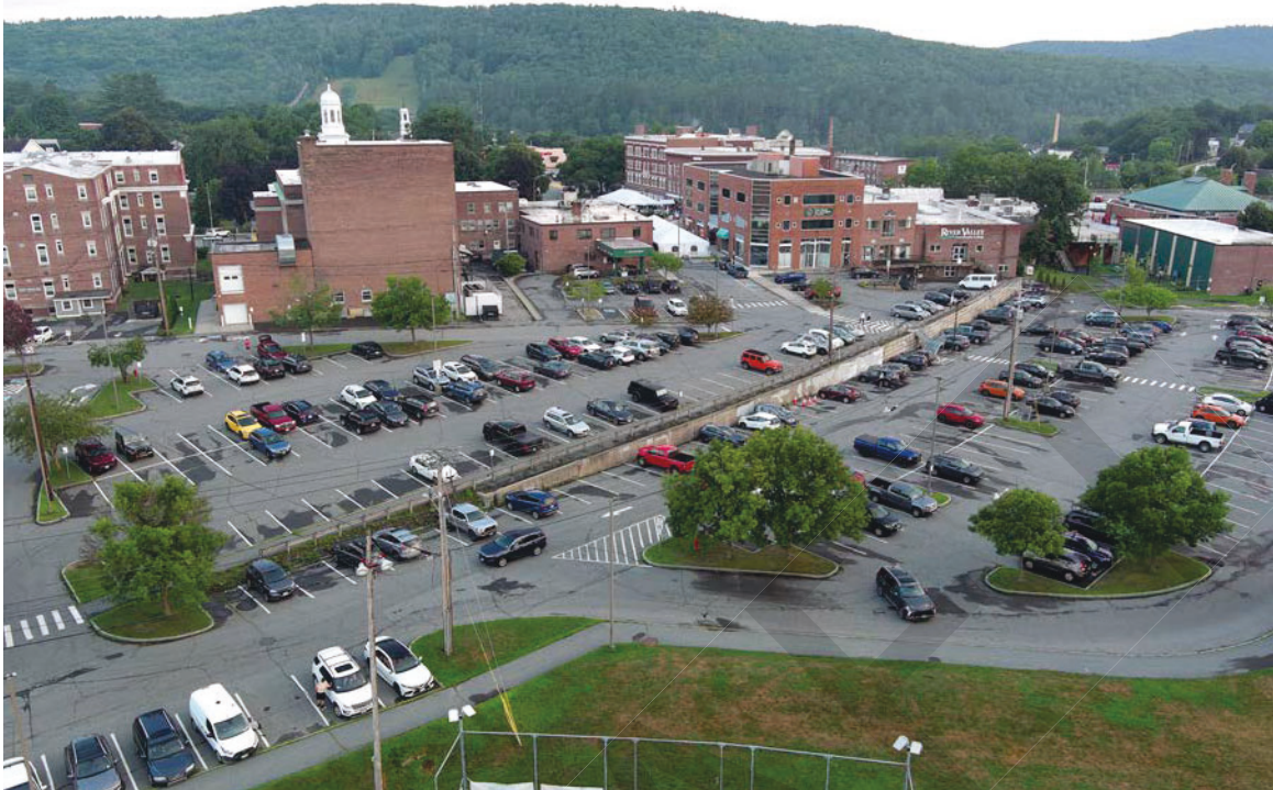
AERIAL VIEW OF SITE LOOKING TOWARD CITY HALL AND COLBURN PARK
