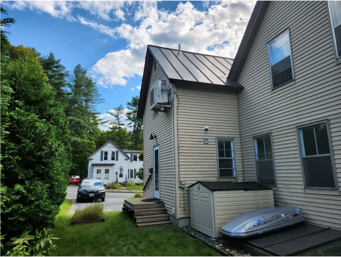
Existing Conditions View from Backyard
