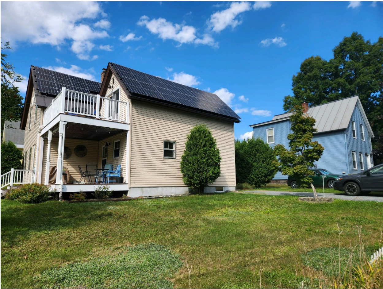
Existing Conditions View from Water-Spring Intersection
