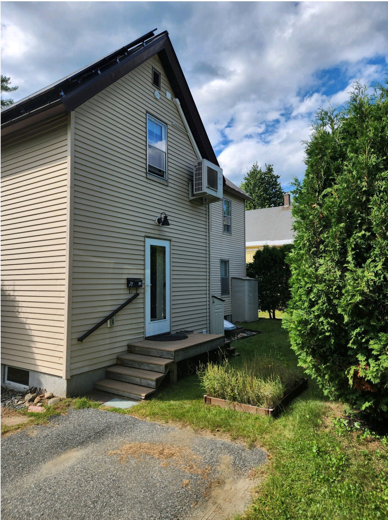
Existing Conditions View from Driveway
