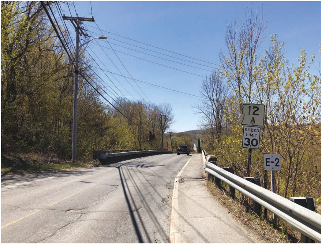
Rte 12A/So Main Street Bridge
