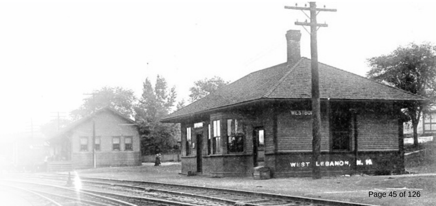
C. 1915 VIEW OF THE FREIGHT HOUSE AND WESTBORO DEPOT, LOOKING NORTH (FROM 2003 WESTBORO RAIL YARD SURVEY)
