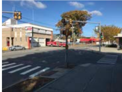
(TOP) EXISTING VIEW OF MAIN STREET AND TRACY STREET INTERSECTION;
