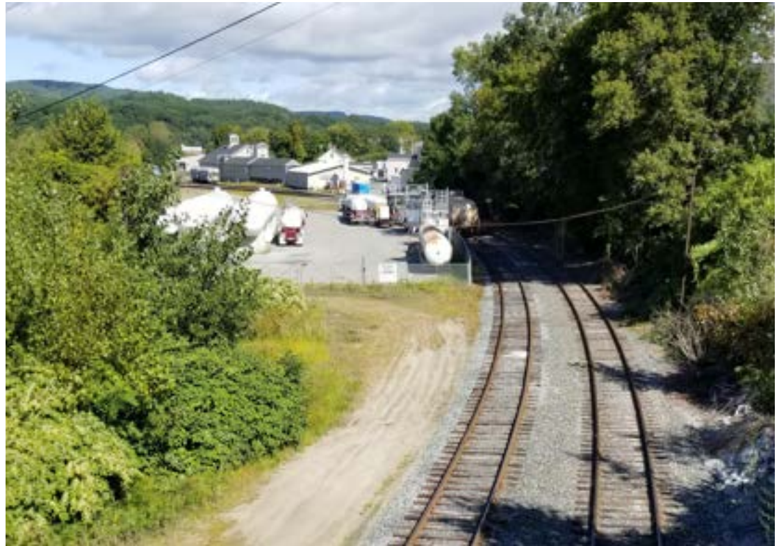
VIEW OF WESTBORO YARD LOOKING NORTH FROM S. MAIN STREET
